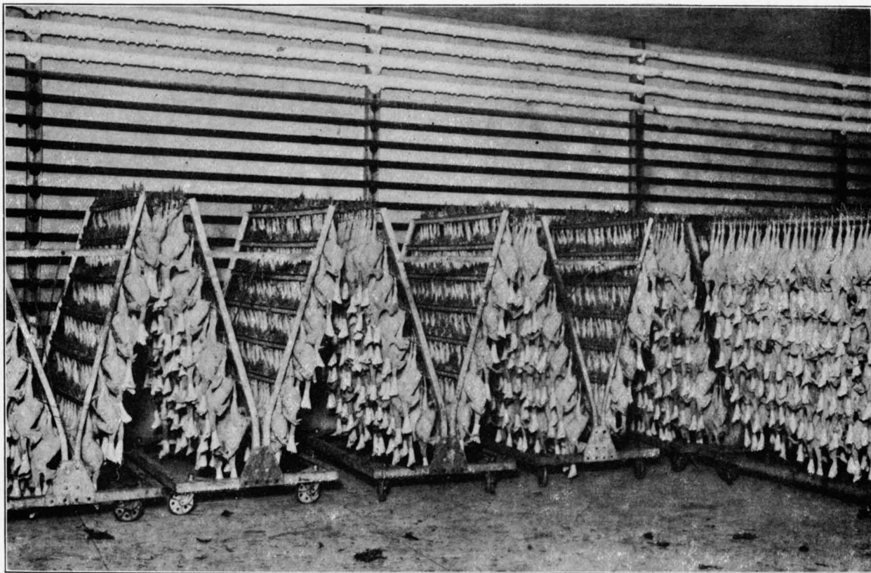
METAL POULTRY-CHILLING RACKS, STANDING IN A MECHANICALLY COOLED CHILL ROOM.
