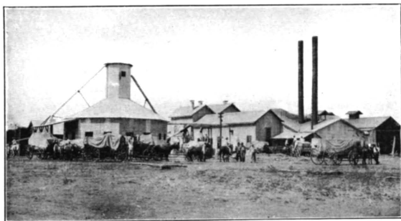
FIG. 2.—TYPICAL COMMERCIAL GIN PLANT IN SOUTHERN TEXAS, SHOWING OCTAGONAL STORAGE HOUSE FOR SEED COTTON, WITH MODERN SYSTEM OF PNEUMATIC UNLOADING AND CONVEYING PIPES.
