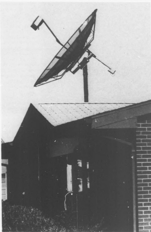
This satellite dish at the County Extension office in Marshalltown, Iowa, was installed on a tall pole beside the building both for better reception and as a security measure against vandalism. Since summer 1986, enough satellite receiving equipment has been installed at county Extension offices throughout the state so that no one has to drive more than 20 minutes to reach an Iowa State University Extension downlink site.
