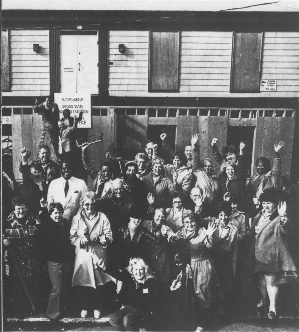
Extension volunteers and staff celebrate the initial construction phase of the new Multnomah County Extension Education Center in Oregon. An aggressive Extension marketing program based on "raised visibility" brought about county funding for the center and a bright image.
