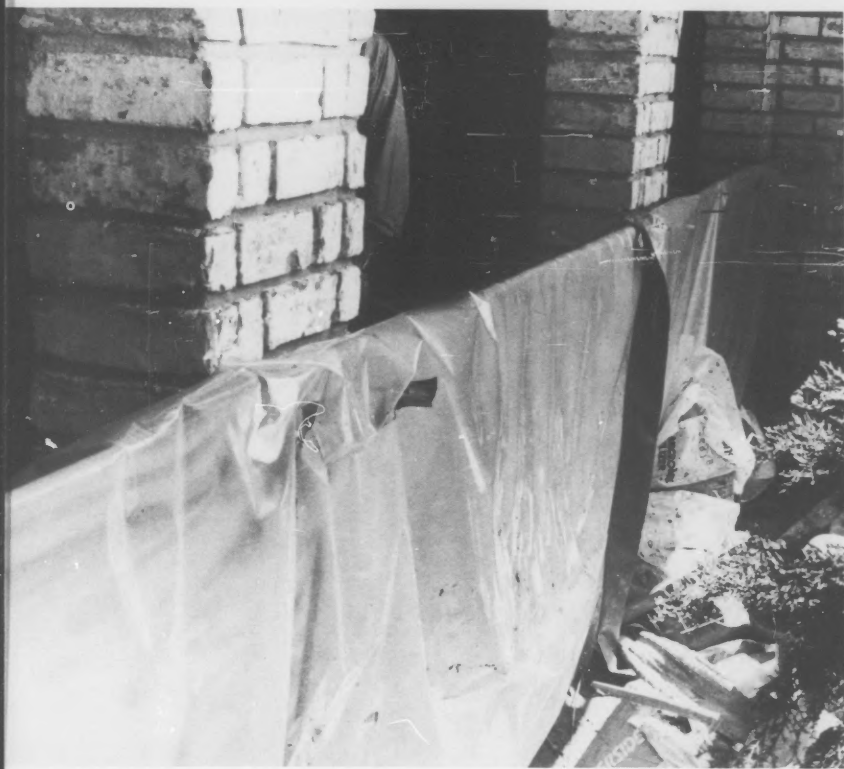
Three 100-foot rolls of polyethylene plastic sheeting wrapped the McManus home against floods that ravaged southeast Louisiana earlier this year.
