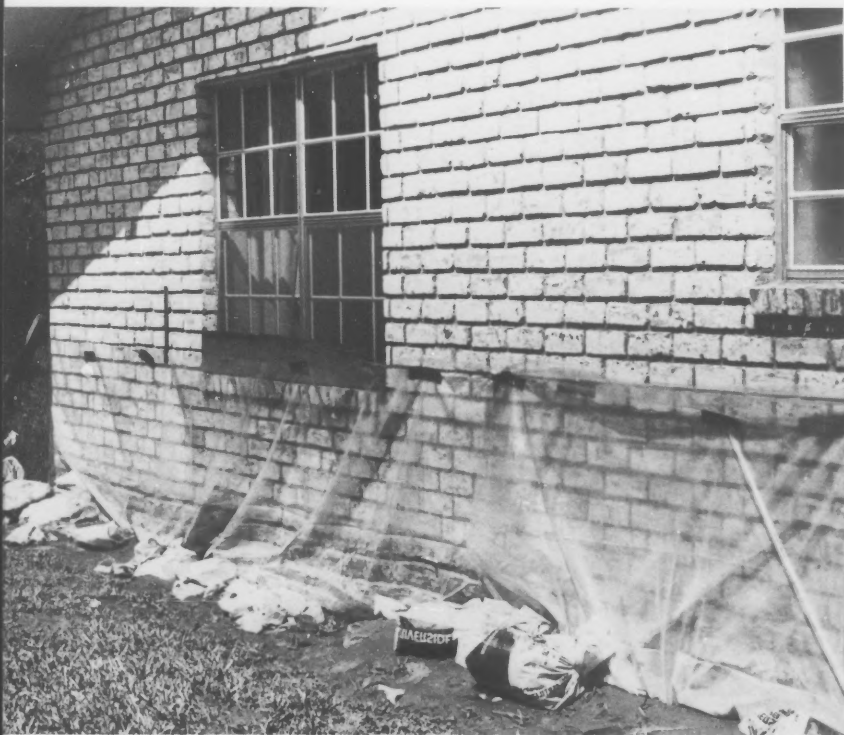
The polyethylene plastic sheeting around the McManus home was attached to the outside walls with masonry nails.
