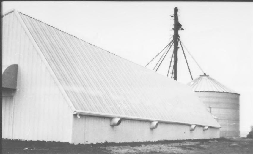
This solar-heated unit in Illinois is used as a swine farrowing house and nursery building. Solar-heated air is also used for drying grain.
