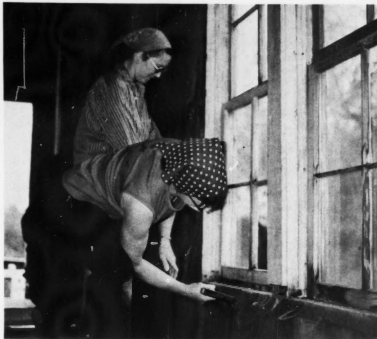
Before nailing on the paneling, workshop participants line the walls with polyethylene.
