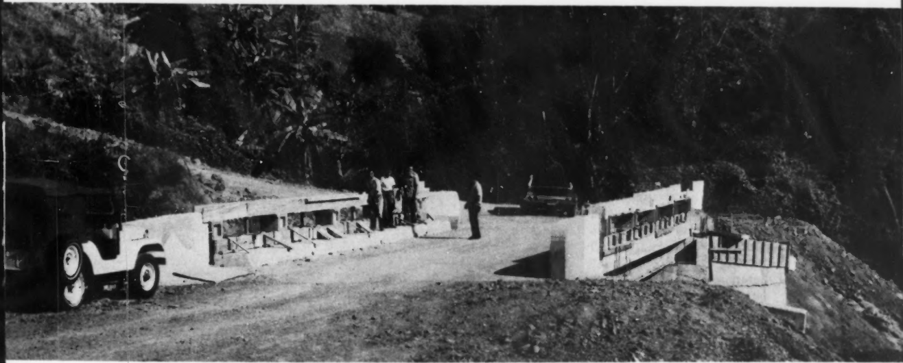
This new bridge joins the once isolated community of Cerro Gordo with the outside world.
