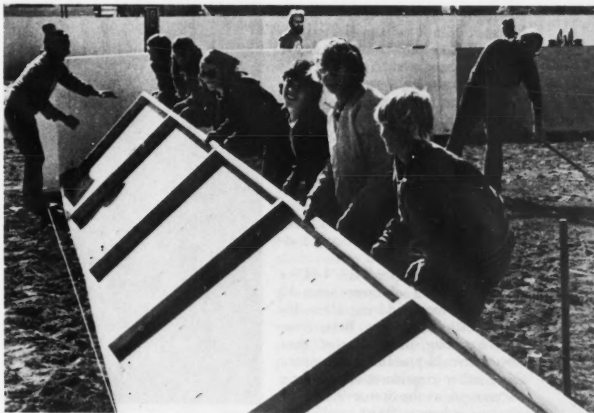
Erecting the hockey boards around the ice rink took a lot of effort and cooperation.
