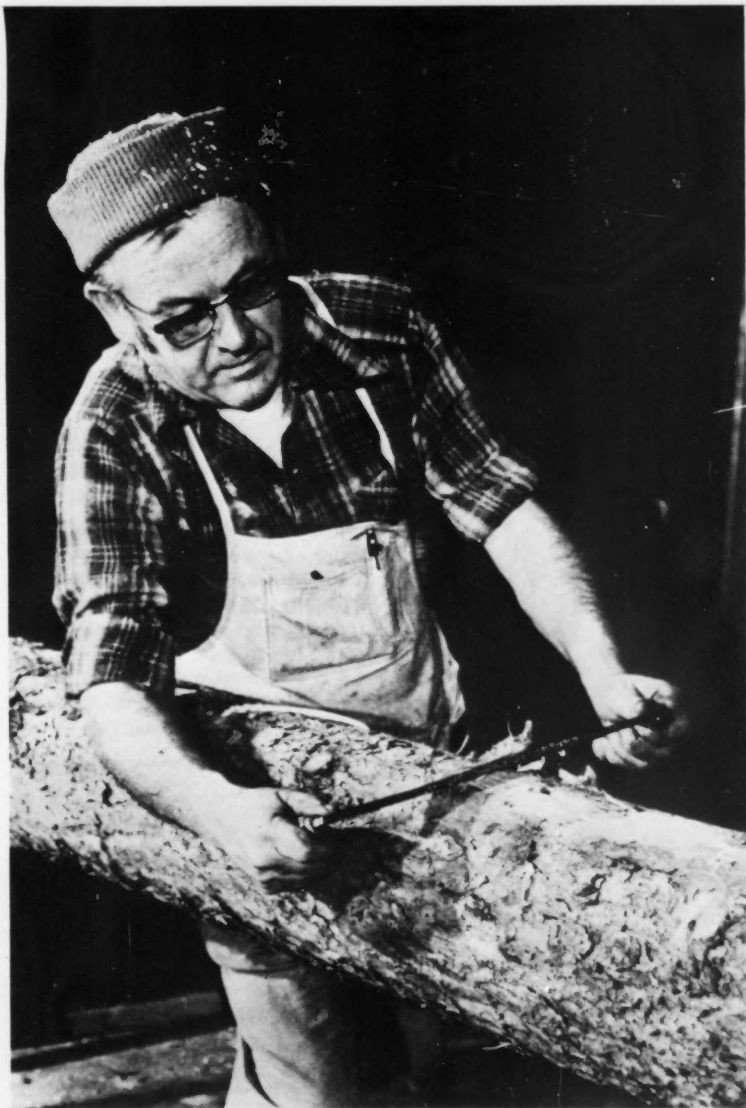
One of the hard-labor aspects of log cabin building is peeling the logs. Here Carlson demonstrates the use of a draw knife in an Alaskan log cabin workshop.
