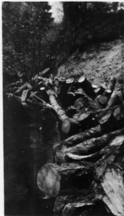
Erosion of the bank above has been stopped with a log jam revetment. Extension refers property owners to the Michigan Department of Natural Resources for technical assistance on such projects.
