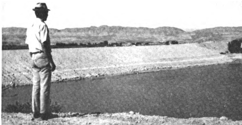
County Agent Ferren Bunker, coordinator of the project to enlarge the Bowman Reservoir, looks at the results of the effort. The dam was raised 22 feet above the original.
