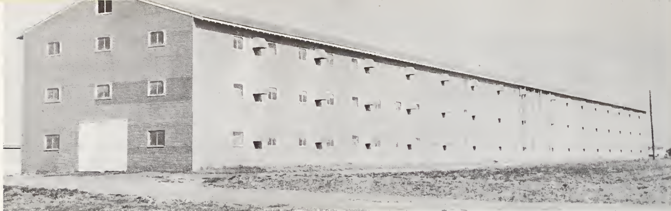
Modernizing facilities was a major method used by Delmarva poultrymen to improve their competitive position. Above is a modern chick motel with central heat, insulation, mechanical ventilation, and auger type mechanical feeders. At right, Ed Ralph, associate county agent of Sussex County, inspects one of the ventilating fans in a broiler house under construction.
