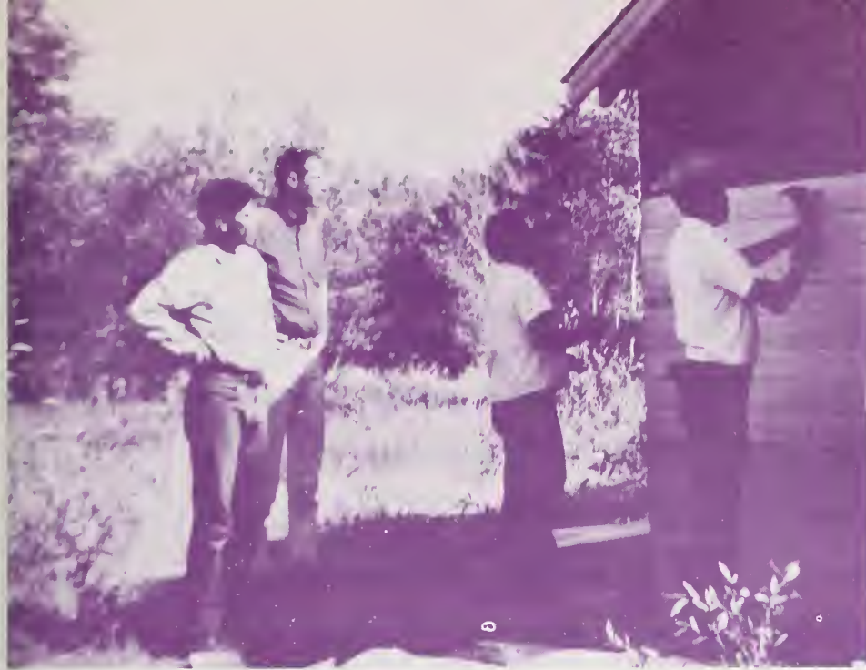
As the agent supervises, the men apply siding to the structure built during the 3-day self-help housing workshop.
