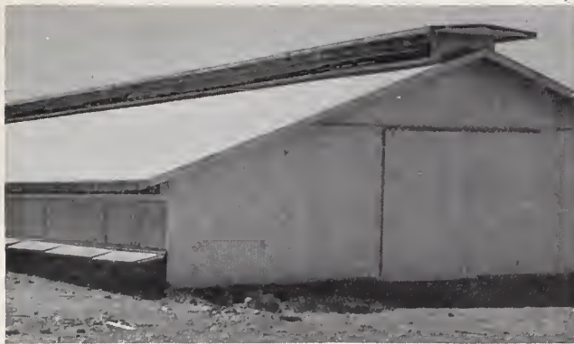
A 40' x 400' broiler house utilizing conventional construction and natural ventilation. The building incorporates continuous ridge vents with continuous floor level ventilation and makes use of adjustable sidewall curtains.
