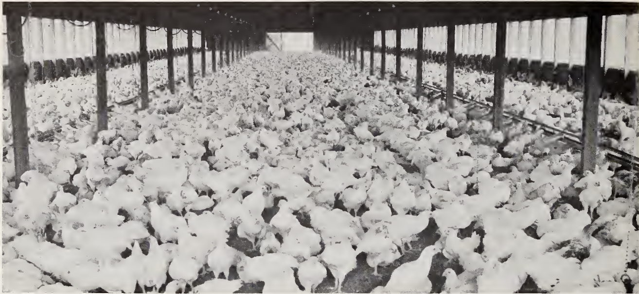
This broiler house has adjustable sidewall curtains. It incorporates natural ventilation in summer and winter.
