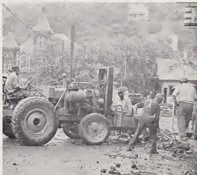
Cleaning debris from US Highway 250 after 1948 flood.
