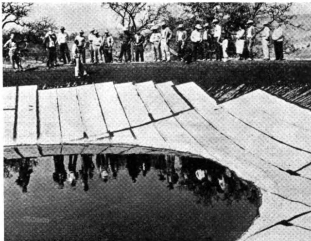
Group approach to a community problem is evident in this cooperative tour with SCS on lining of water storage range reservoirs.
