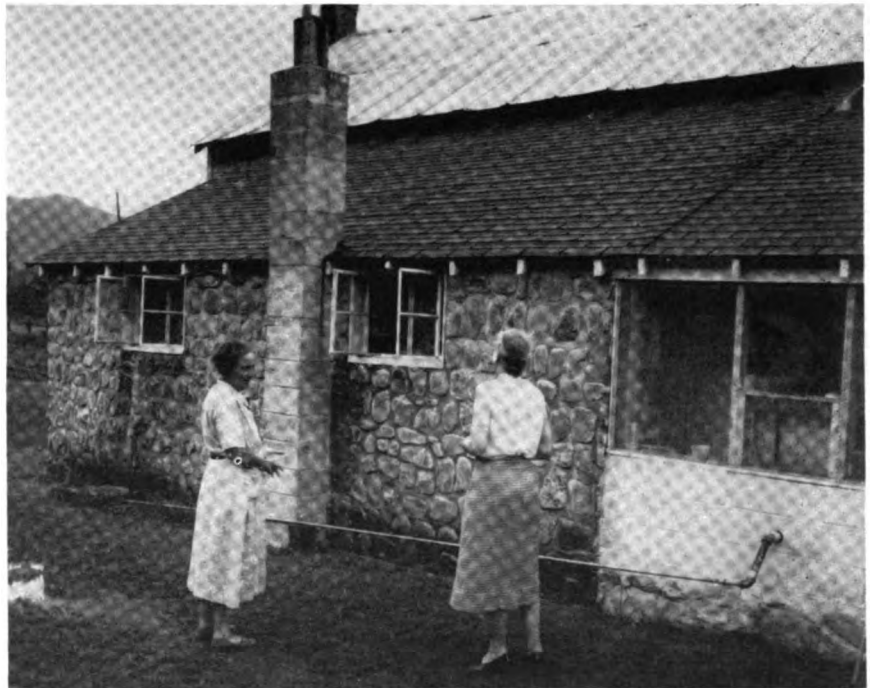
Mrs. Thomas Martin (left), rural homemaker of Montgomery County, and Mrs. Kate E. Hoge, county home demonstration agent, are looking over the stone work which Mr. Martin, himself, put on the outside of their old pre-Civil War house as part of their long-range improvement plan.
