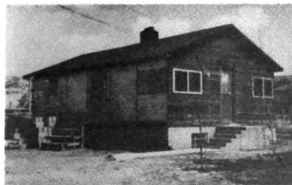
Improvements in Melvin Mellor home, Sanpete County, Utah, are clearly evident in these before and after photos. House remodeling
