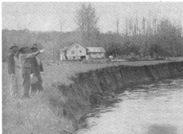
When river bank protection is missing, acres of good loam soil are washed away during spring floods.
