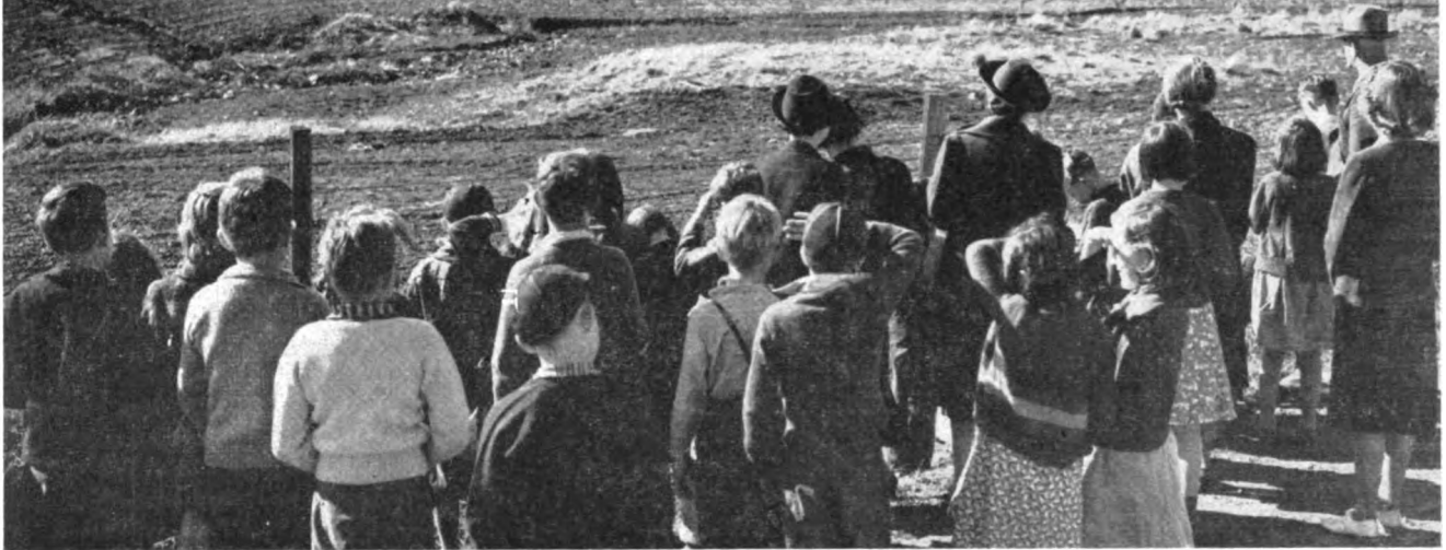
Visible evidence of soil erosion
