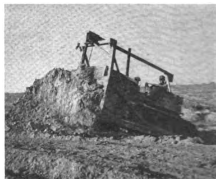
Excavating for a pond.
