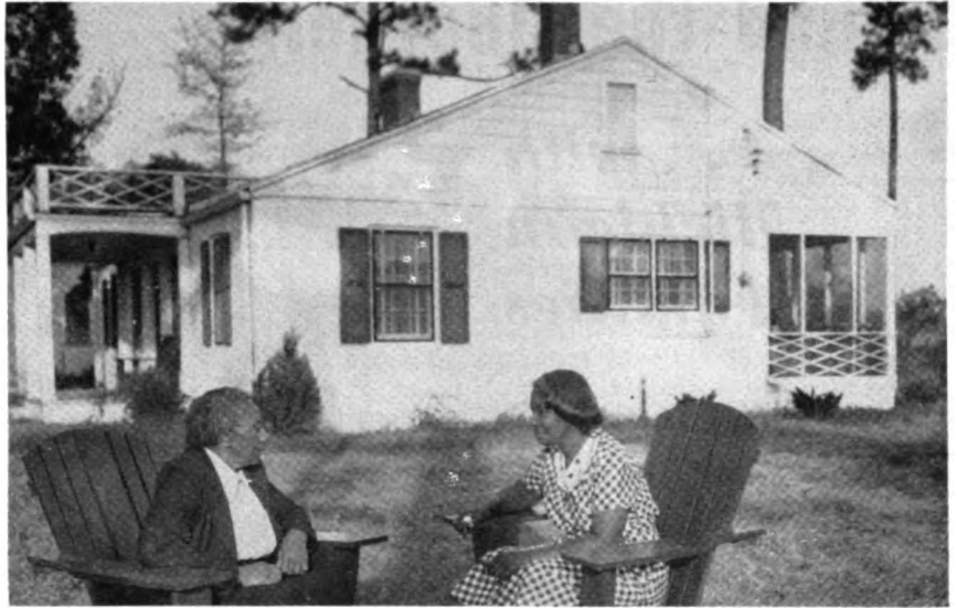
This is the dream house which is changing the face of the South Carolina countryside and two of the vacationers taking it easy on the lawn. When a house is planned and built for efficiency and comfort, the work doesn't take long.
