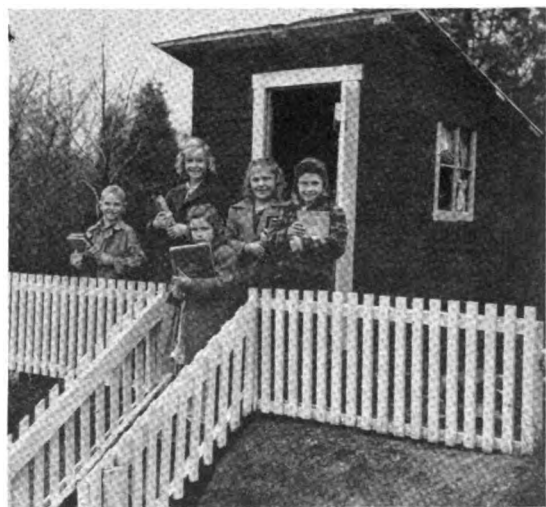
Here's what a community built for its school children—school bus waiting stations with safety chutes for loading and unloading the children to prevent their scattering.
