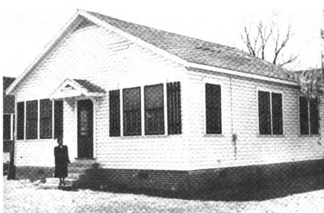
Washington County Extension Building at Greenville, Miss., has kitchen, meeting room, and office space.
