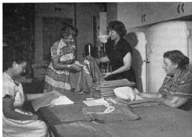
Looking over the progress they had made.
