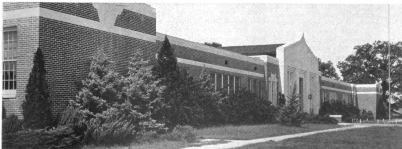
One of the principal points of interest in this Mississippi town is this beautifully landscaped rural high school.
