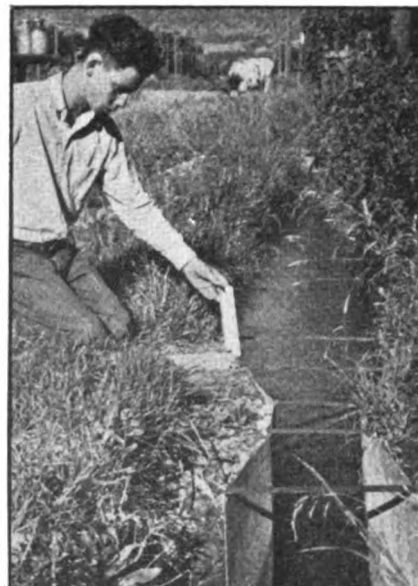
Taking a reading on one of the weirs used in the Utah irrigation program.
