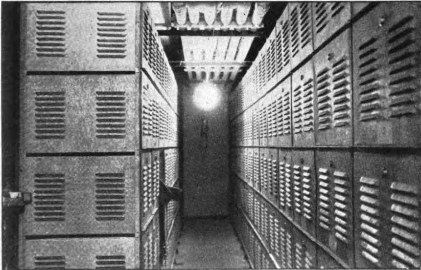
Locker storage room of a meat plant at Litchfield, Minn. In this room the cuts of meat in labeled, bloodproof packages, are stored at a temperature of 5° or 6° below zero. Farmers may enter the room to get any cut of meat they desire.
