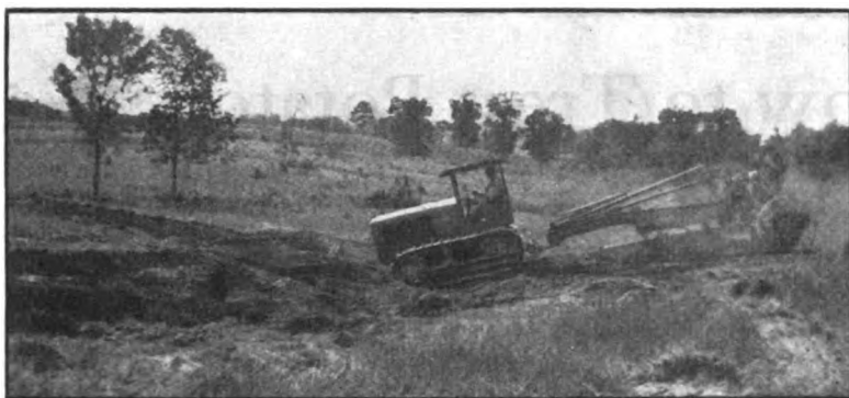
The grader and cat in operation.
