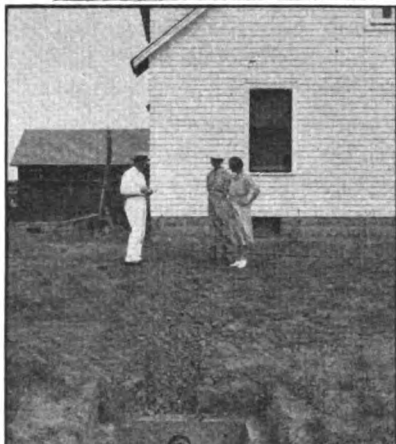
A Kansas farmer constructs a septic tank.
