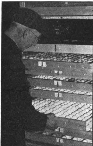
A huge electric incubator near Morristown, N. Y., automatically maintains the most efficient temperature and moisture conditions.
