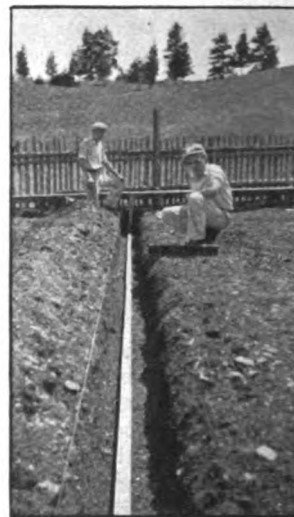
Two members of the Mortgage Lifters' 4-H Garden Club, Lewis and Clark County, Mont., laying the first lath tile subirrigation system in the county.
