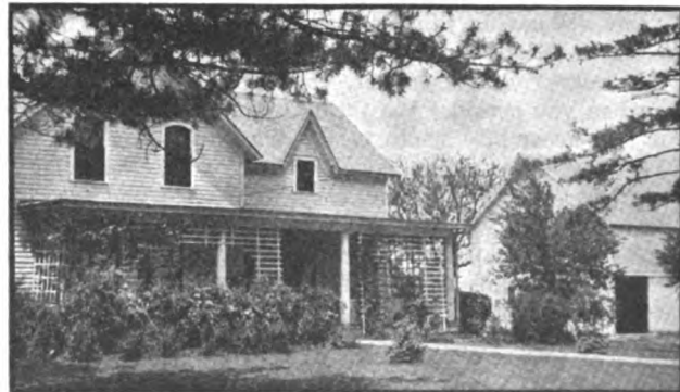
Clean paint, clean yard, and landscaping add to the home appeal of Harry Wade's farm home.
