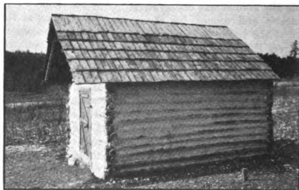
A log storage house, costing 87 cents in cash, erected in Saline County, Ark. More than 1,063 such storage houses were put up in 56 Arkansas counties from Extension Service plans.
