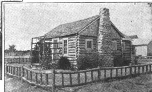
Prairieville (Tex.) Community House is built of native logs cut in a nearby woods and put up by the men of the community.
