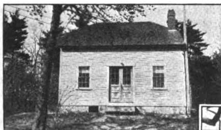
(Left) The Damariscotta (Maine) Community House is an old schoolhouse remodeled by the men of the community working 2 nights a week. It boasts a fine kitchen and is built to withstand the coldest Maine winter.
