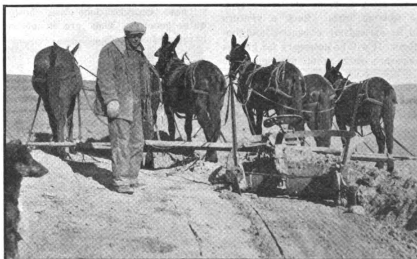
The terracing machine owned by the Webster County Farm Bureau is lent to farmers as part of the campaign to check erosion and conserve soil fertility. Here it is seen in action on one of the 75 farms that have terraces.
