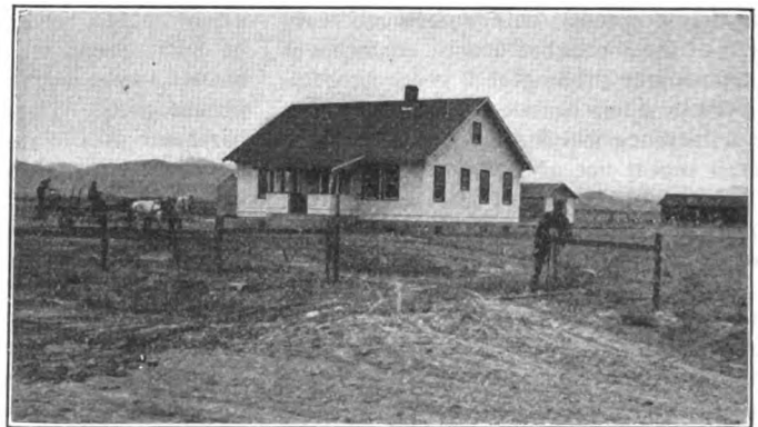
Grading the driveway to the community house of the Willwood irrigation project as a demonstration in home improvement.
