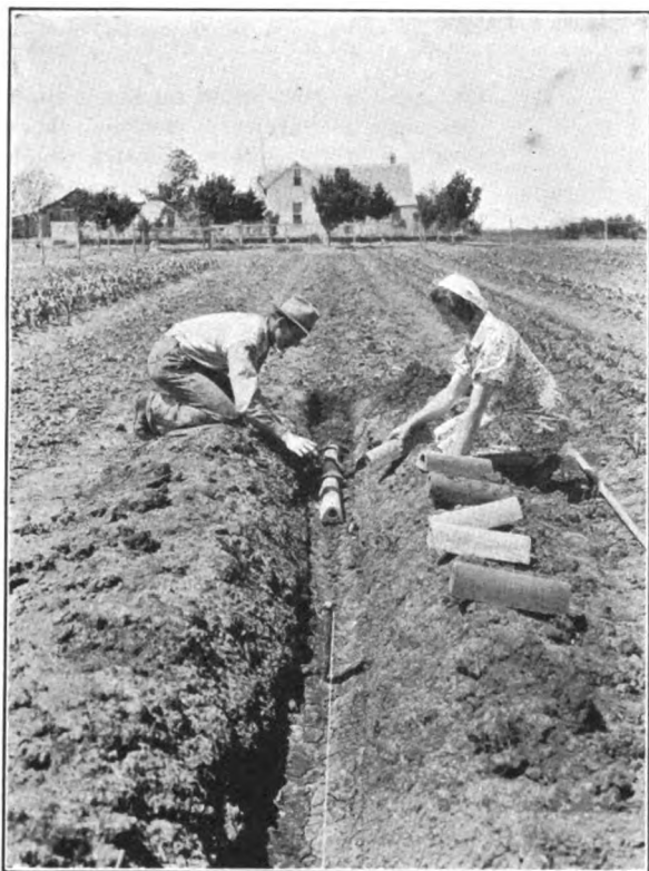
Subsoil irrigation with home-made tile has saved many a Texas garden
