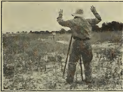
Laying lines for a new terrace
