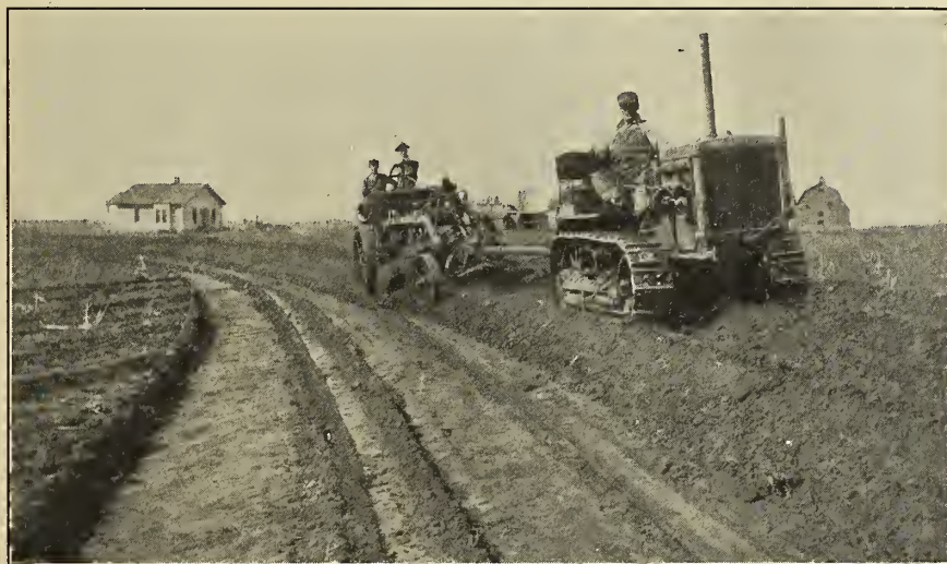
Using county road machinery to construct terraces in Seminole County, Okla.
