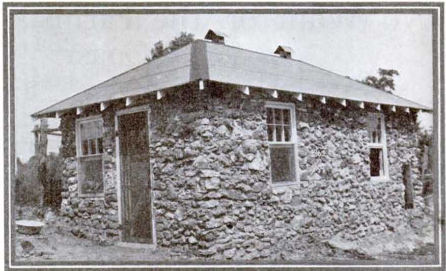
This milk house was built of cobblestones at a cost of $75
